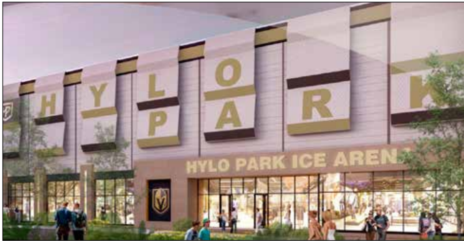
The Hylo Park Ice Rink, which closed recently for renovation, isn't scheduled to re-open for 12-14 months. (Agora Realty)
